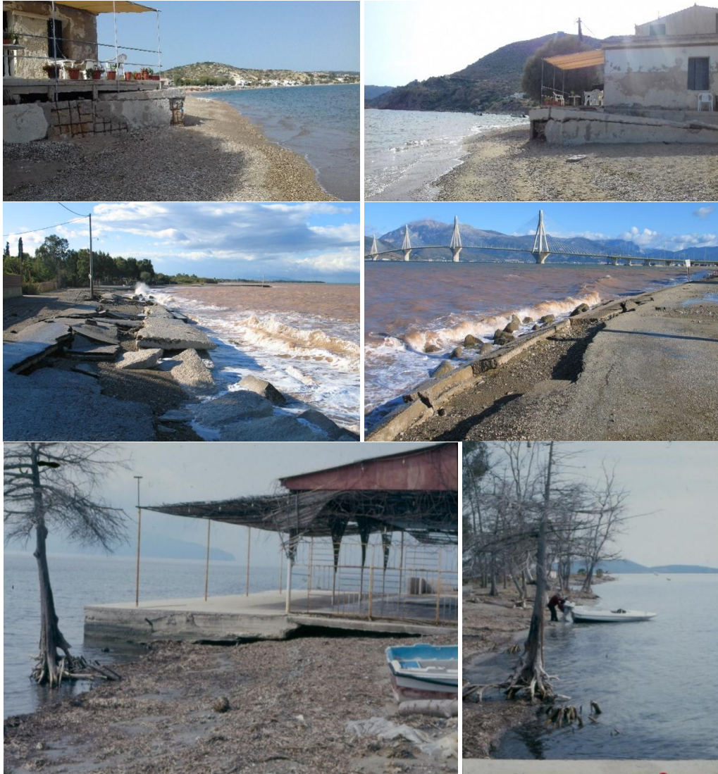
Fig. 1. Man-made interventions combined with climate changes and the expected sea-level rise affect the coastal zone. Some examples of coastal erosion-shoreline retreat, along the Greek coast: Figures 1a-b: Chios island-Komi, 2017, Damages to a house in Komi beach, caused by coastal erosion, Chios island, Greece. Figures 1c-d: Patra-Rio, 2009, Damages to sea front road in Rio, caused by a storm wave event on Rio, Patra, Greece. Figures 1e-f: Amvrakikos Gulf-Preveza, 1990, Coastal erosion and shoreline retreat in the coastal zone of the Preveza city (Photos by Mertzanis A.)
