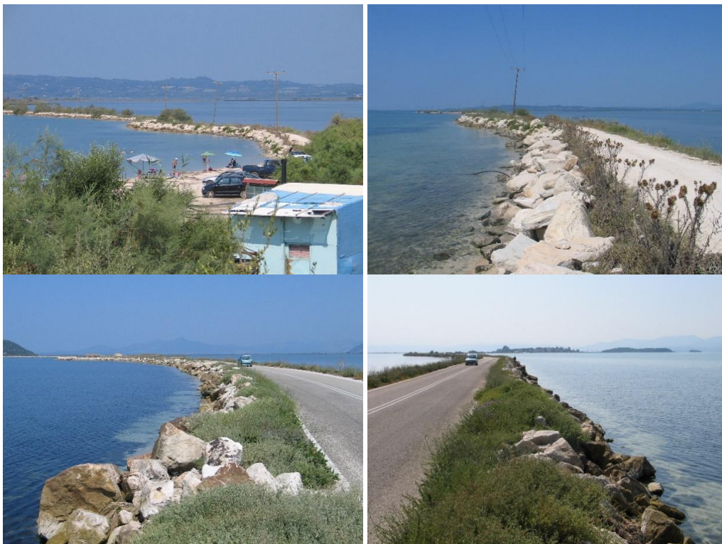
Fig. 5. In the Delta of the Arachthos river, since the construction of upstream dams in the Arachthos river basin, the deltaic shoreline, sandy coasts and the sand barrier which connects Koronisia with Fidokastro, are subject to erosion processes. The thin sand barrier between the Tsoukalio lagoon-Amvrakikos Gulf (Fotos 5a-b) as well Logarou lagoon -and Amvrakikos Gulf (Fotos 5c-d), being under erosion by wave action, but are supported by coastal protection works along the shoreline (rock armour, riprap, etc.)(Photos by Mertzani As.-August 2019)
