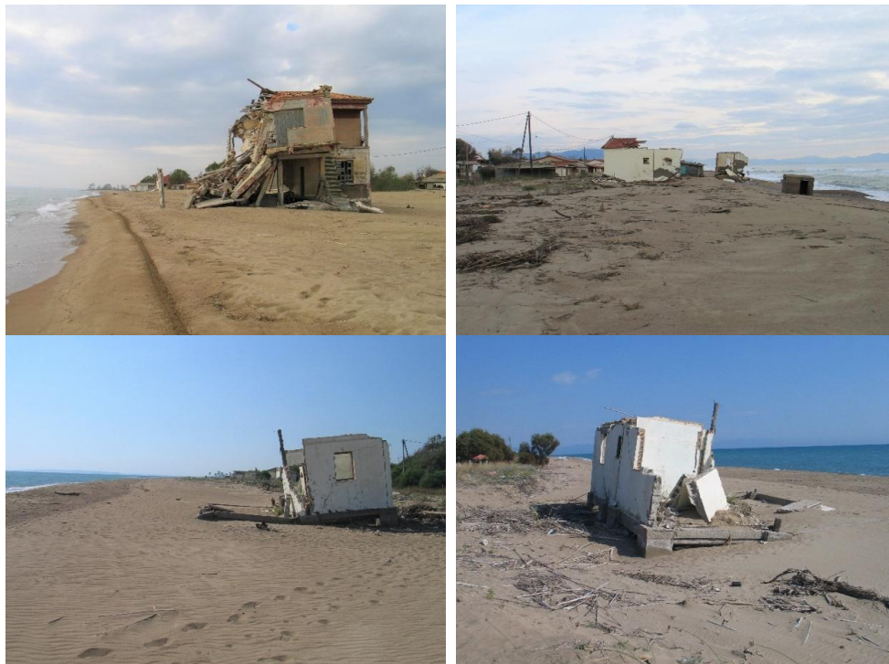
Fig. 8. Difference between the year 2010-11 and 2019 of the Deltaic coastline retreat in the River Alfeios mouth area due to dam construction. Coastal erosion in Paralia Epitalion (Epitalion beach in the south-east of the estuaries of Alfeios river), results in damage or loss of houses and other coastal structures (Kyparissiakos Gulf-Greece). The coastal area of Paralia Epitalion during 2010 (December 2010) and 2011 (March 2011), is shown in the figures 8a and 8b. The same location during 2019 (August 2019), is shown in the figures 8c and 8d. (Photos by Mertzanis A.)
