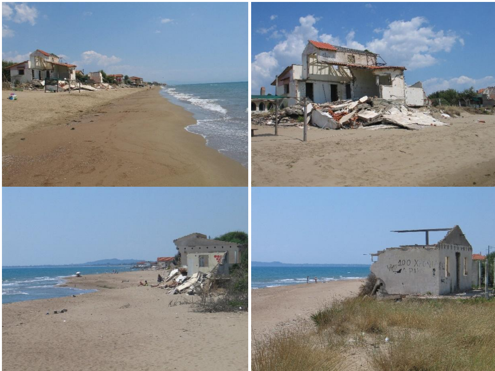
Fig. 3. Deltaic coastline retreat on the River Alfeios mouth area due to dam construction. Coastal erosion in the Spiatzia beach (in the north-west of the estuaries of Alfeios river), results in damage or loss of houses and other coastal structures (Kyparissiakos Gulf-Greece). The area most affected by coastal erosion is the deltaic coast of the Alfeios river, and especially its mouth area, in which has been caused a retreat of the shoreline, of approximately 450 m during recent decades. Coastal erosion and shoreline retreat is expected to increase due to Climate Change and the potential future Sea-level rise (Photos by Mertzanis A.-August 2019)
