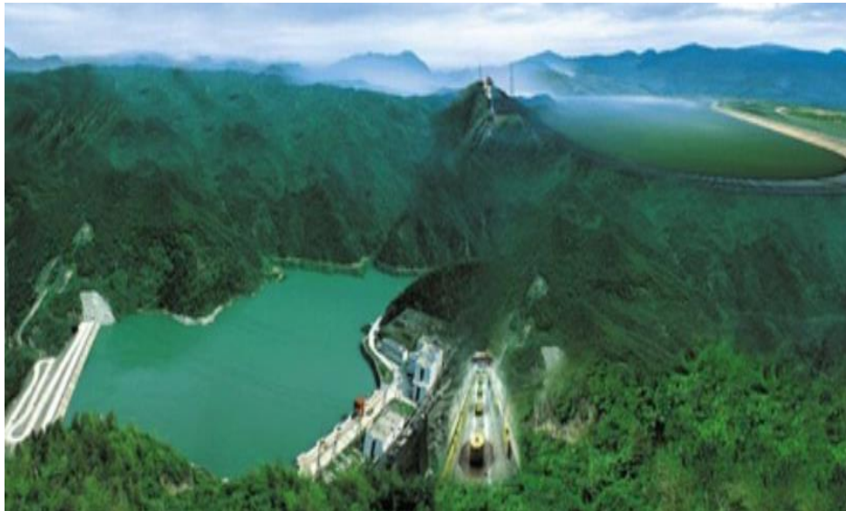
Fig. 2. Pumped storage power station
