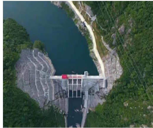
Fig. 4. Hongping pumped storage power station
