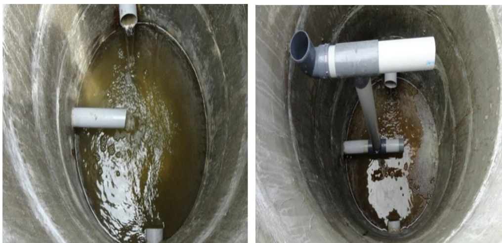
Fig. 2. A view of Conventional and Controlled SSD systems imposed at 50 m lateral spacing at Agricultural Research Station, Gangavathi
