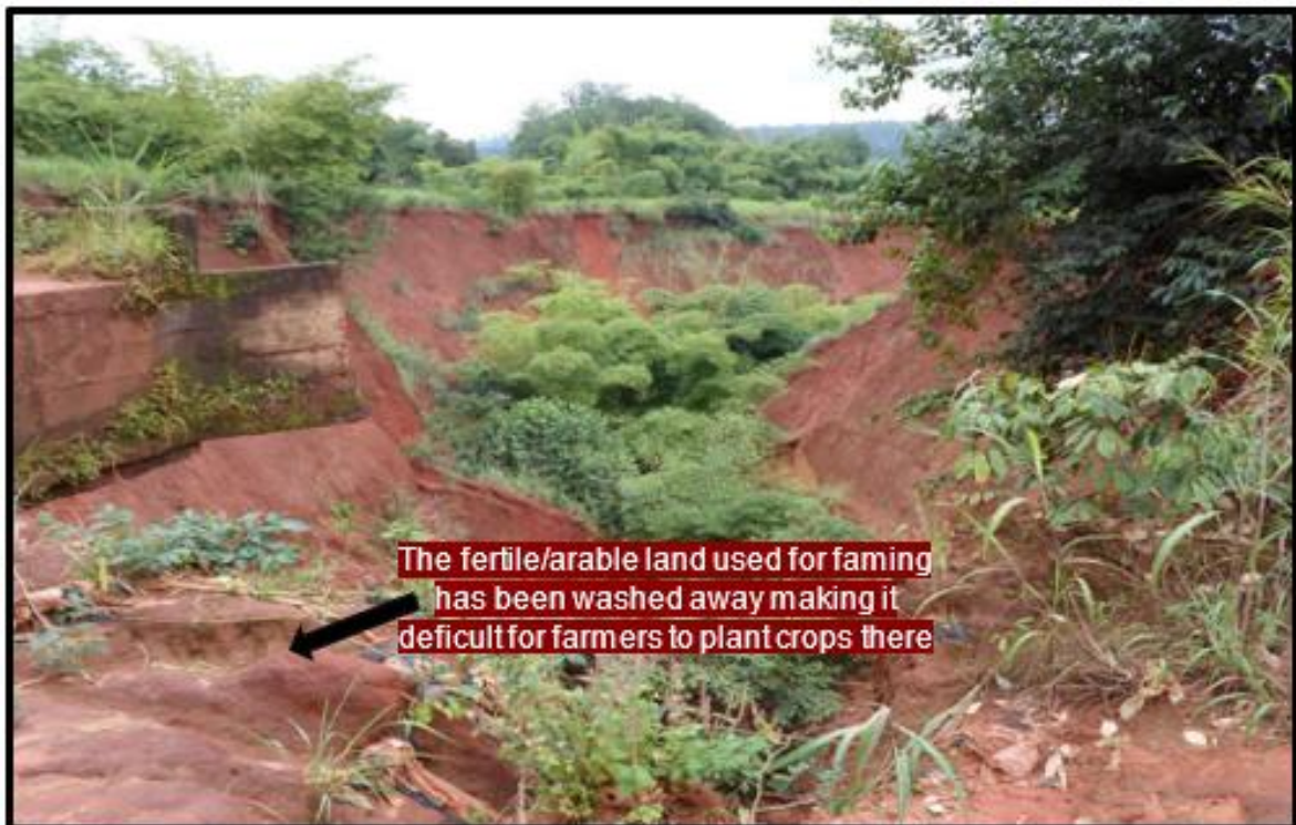
Fig. 7. Gully site at Obinagu village showing loss of productive land [7]
