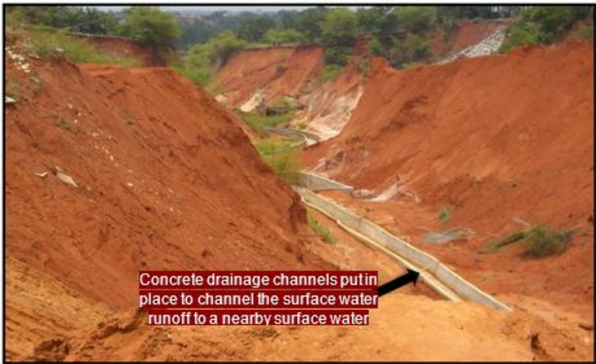
Fig. 8. Control measure put in place to check gully erosion [1]
