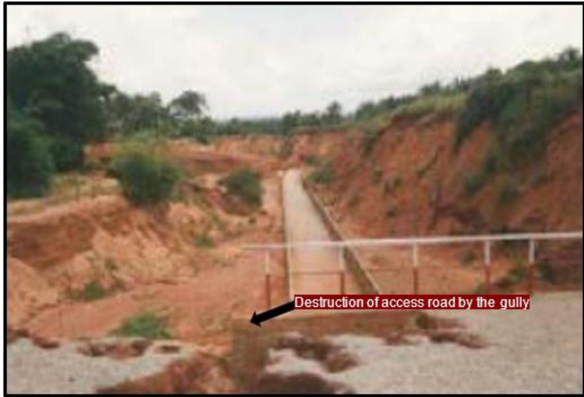
Fig. 6. A Gully Site in Umuchiana, Aguata, showing the dissection of the access road [12]
