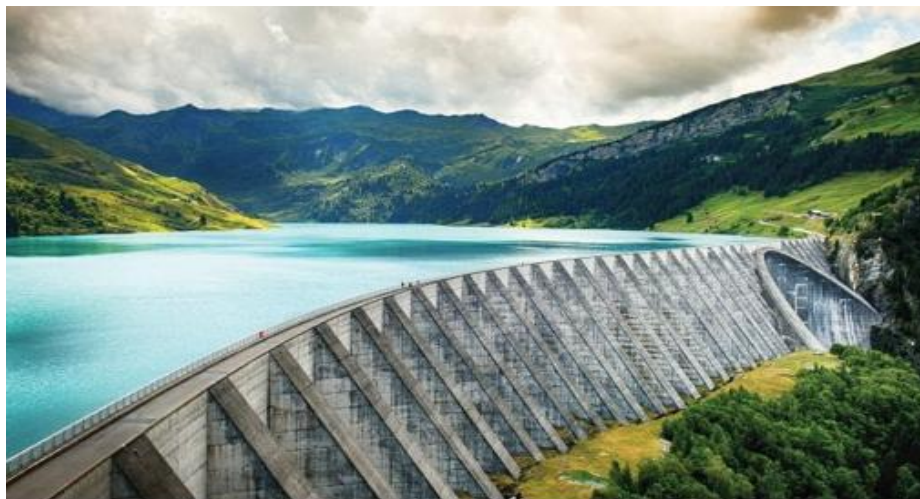
Fig. 15. Roselend Dam, Beaufort, France (source: IRENA , 2018)
