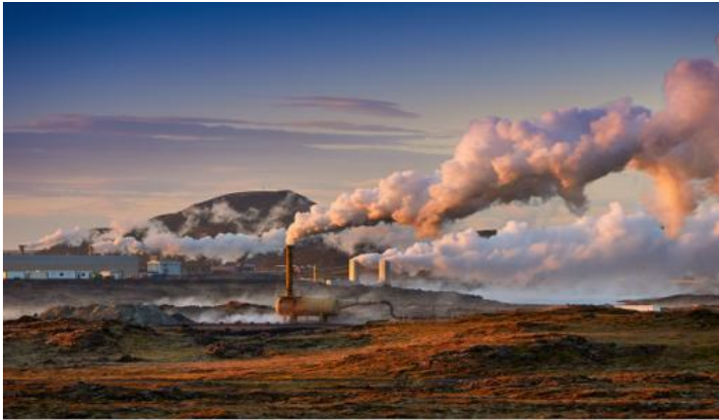
Fig. 17. Geothermal Terminals at Tanzania (source: IRENA, 2019)
