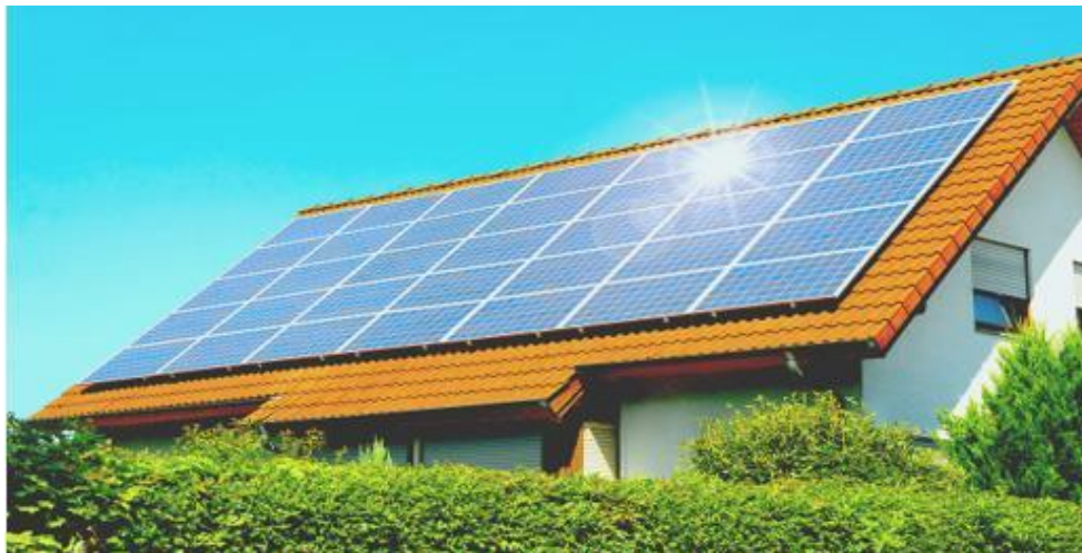
Fig. 13. Roof-mounted solar panels (source: Stern, Burke and Bruns, 2019)
